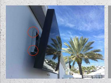
"Mounting onto a brittle concrete surface requires specialized anchoring techniques. This ensures optimal utilization of the superior compressive strength of the material to ensure a robust and safe installation. Improper mounting techniques for concrete surfaces lead to degradation of the concrete support and eventual failure of the mount, which poses a serious safety risk to high traffic areas like ticket windows."
